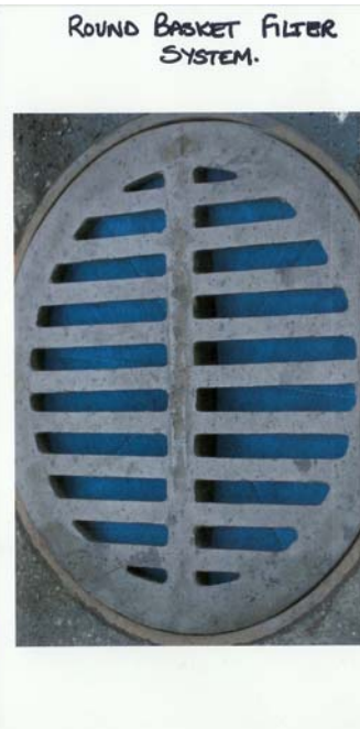
Storm Basket Filter installed
